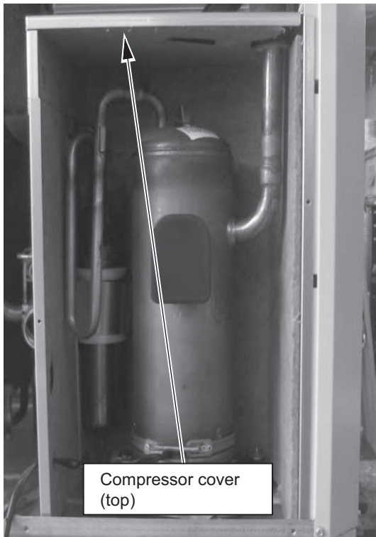
4. Remove the compressor cover (top).
